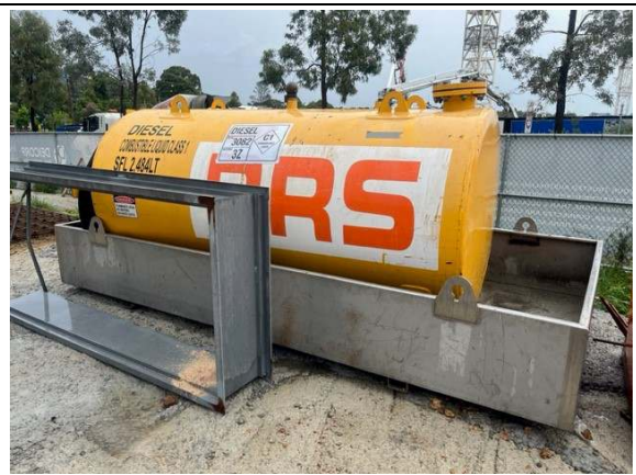
Photos 27 & 28: Diesel and jerry cans of fuel were stored in secondary containment and secure.
